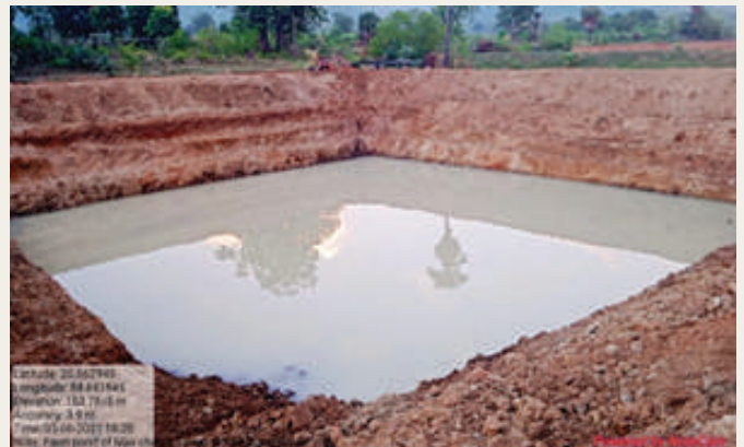
Farm Pond excavated in Kendupati Dalaki VSS in Athamallik Forest Division
